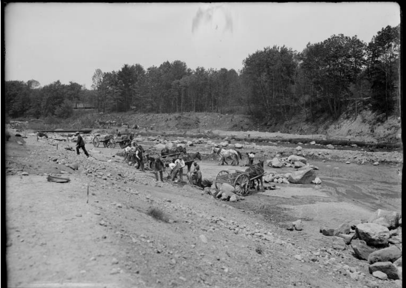
WACH. RES. OAKDALE. IMPROVING QUINEPOXET RIVER CHANNEL. JUNE 2, 1905.
